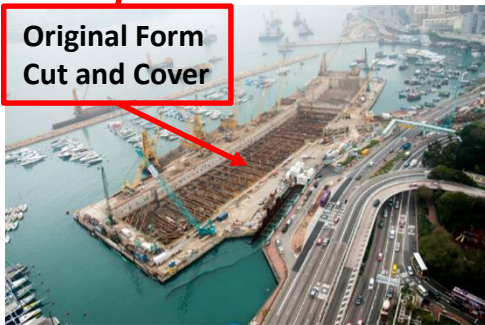
Central Wanchai Bypass (CWB) Under Construction
