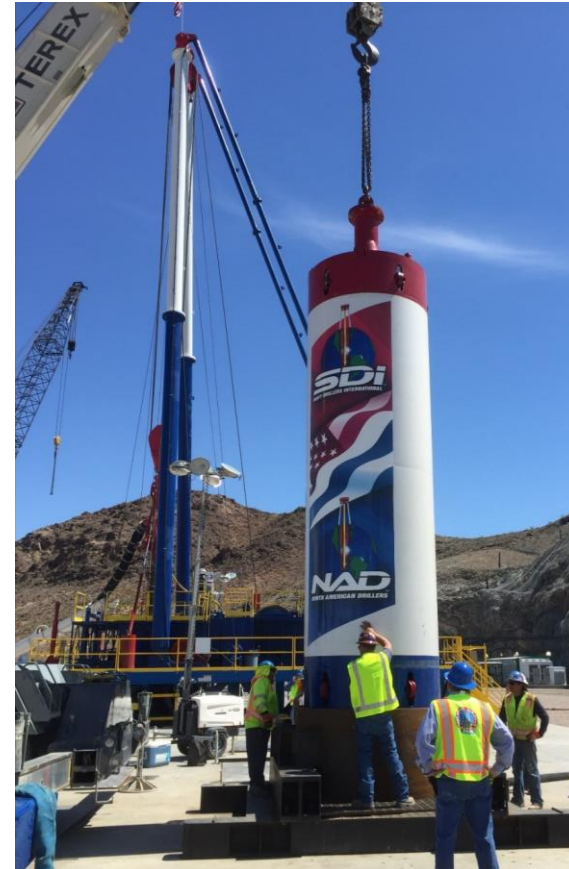
Mandrel (Survey Alignment)
