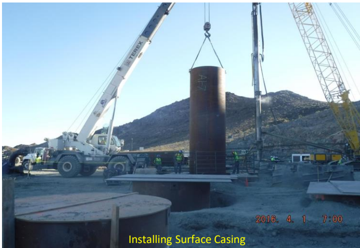
Surface Casing Excavation
