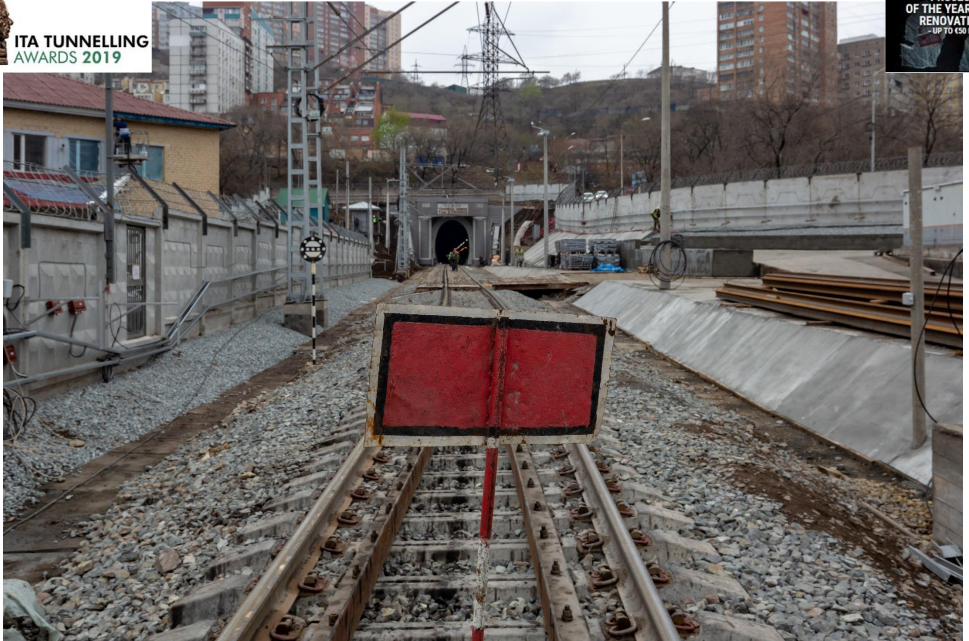
South portal of the tunnel
