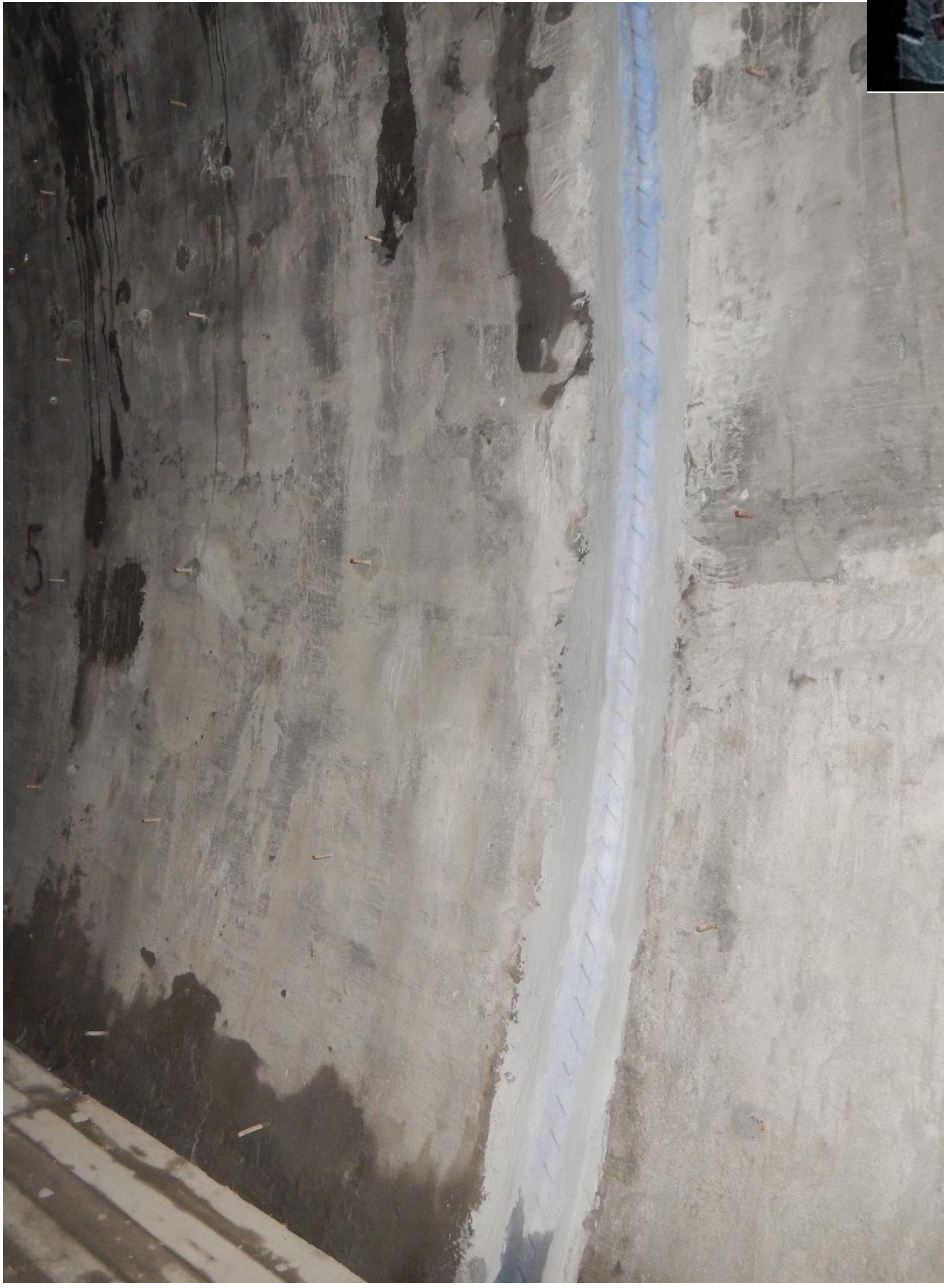
Sealing of expansion joints
