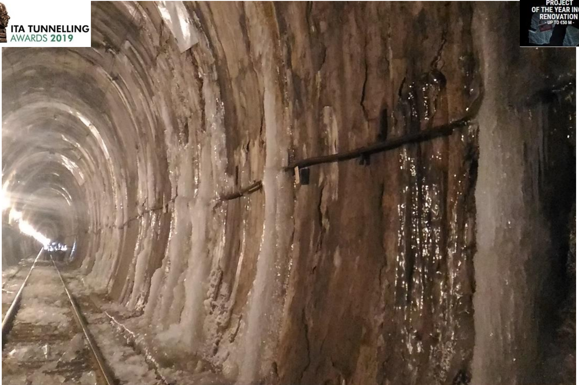
Aufeis formation in the tunnel
