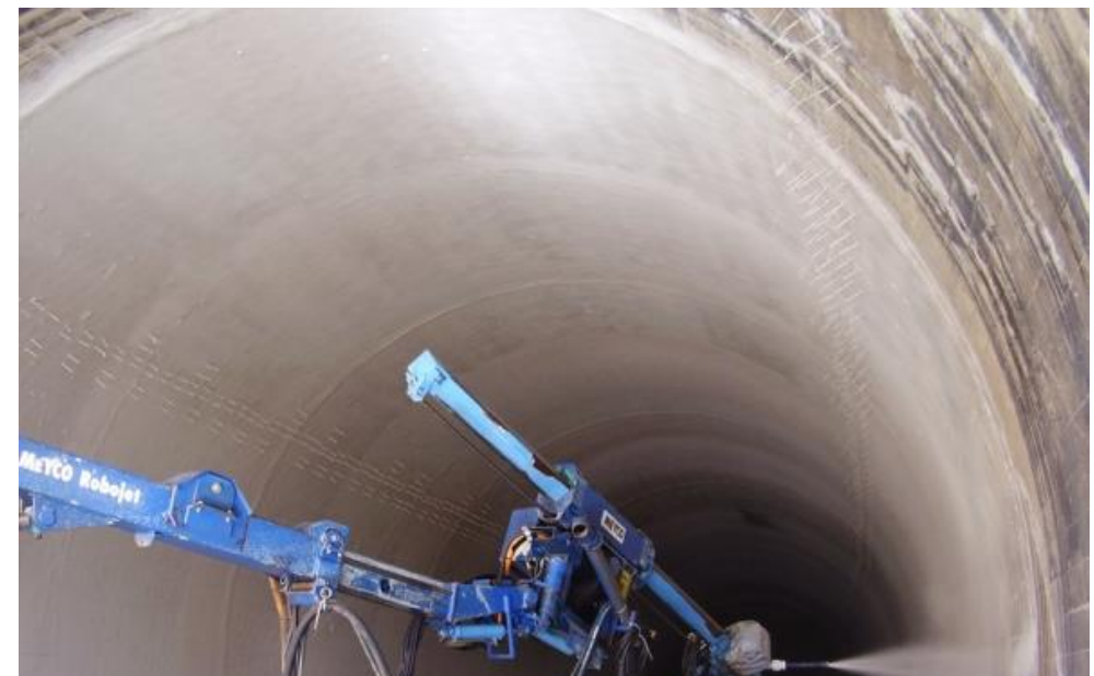
JSC Mosmetrostroy, Modernization of Vladivostok Tunnel of Far Eastern Railway
