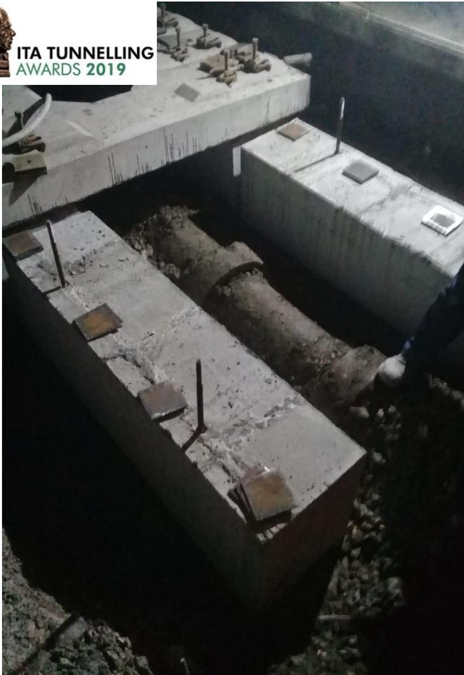
Foundation preparation for track bed structure
