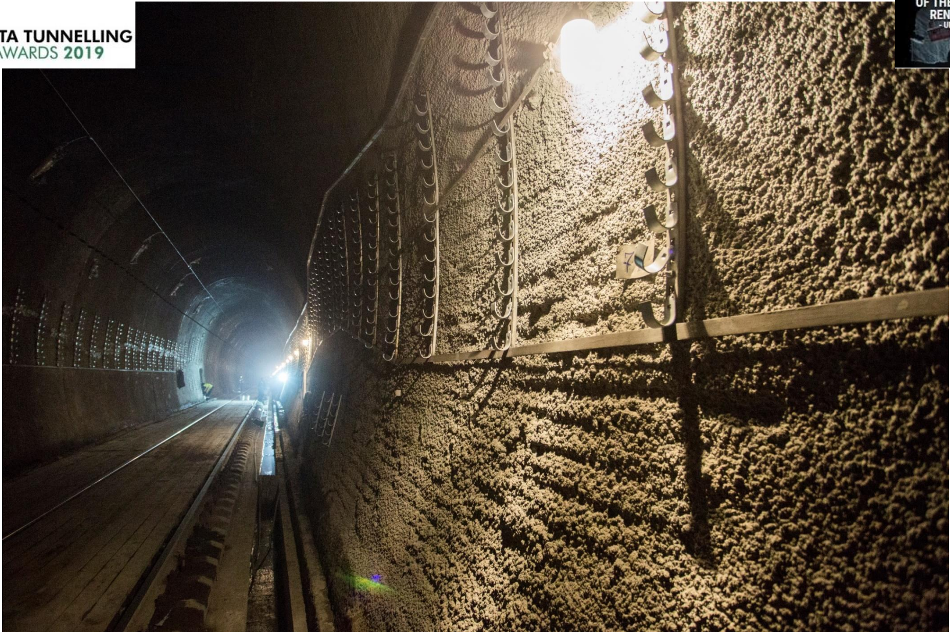
Condition of the tunnel lining after modernization
