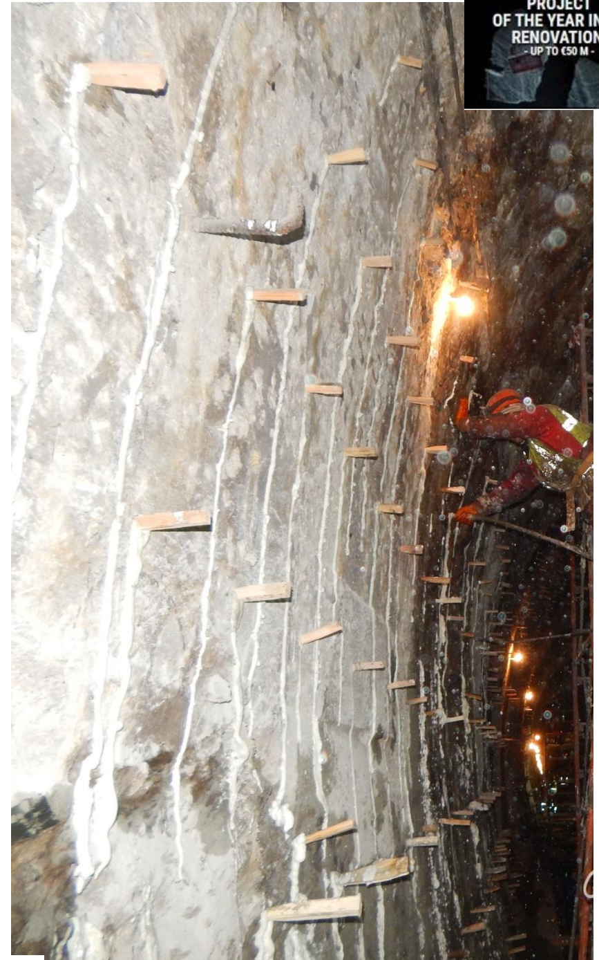
JSC Mosmetrostroy, Modernization of Vladivostok Tunnel of Far Eastern Railway
