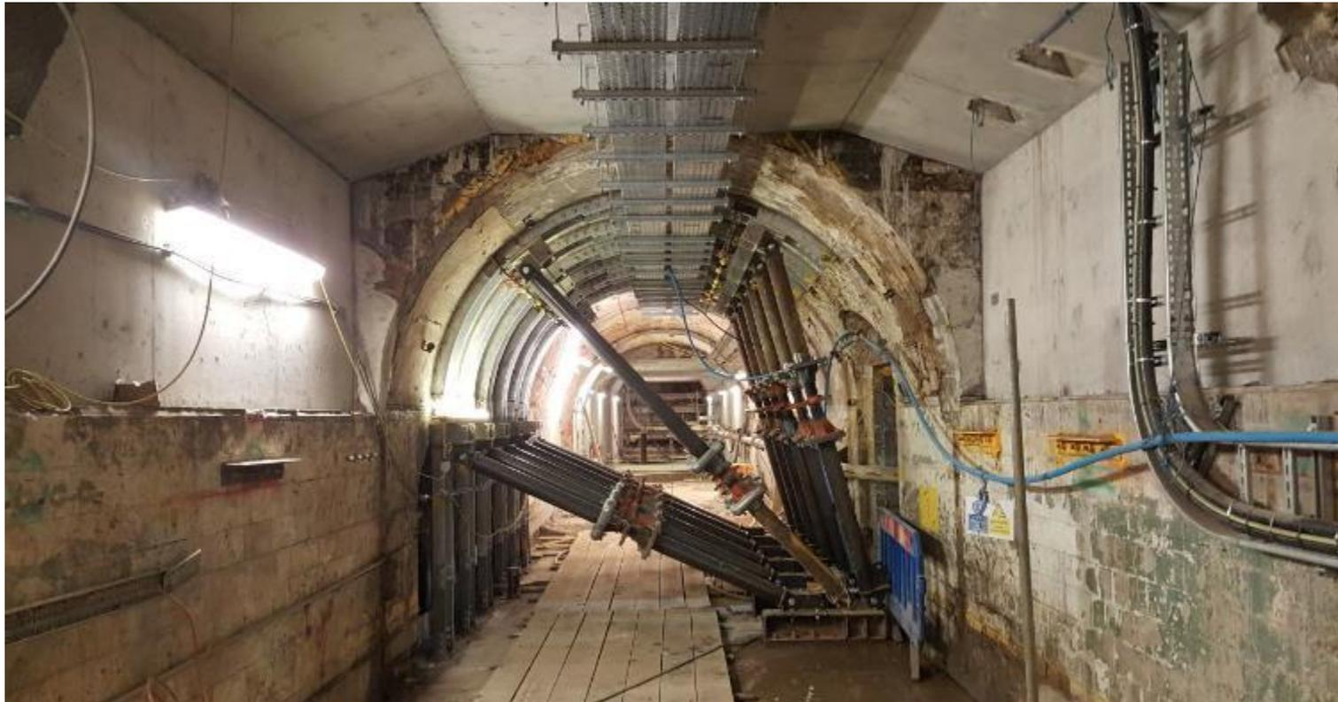
**Innovative temporary & permanent masonry tunnel support shown in temporary support condition prior to formation of new opening**
