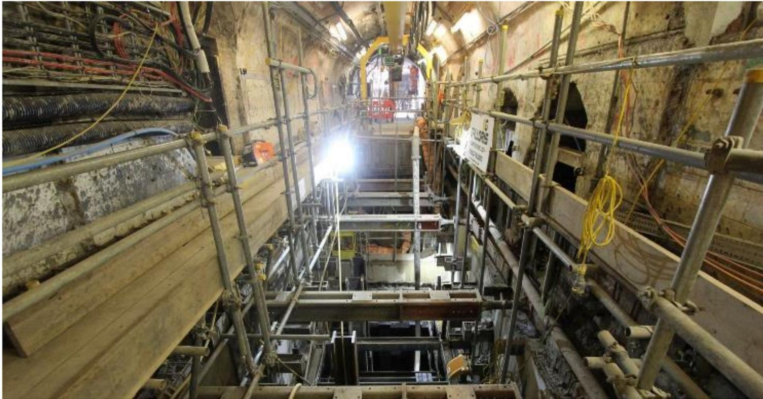
**Underpinning of distressed dis-used passageway between the two Underground Platform tunnels to allow new opening and undermining to form a new access to new lift shaft**
