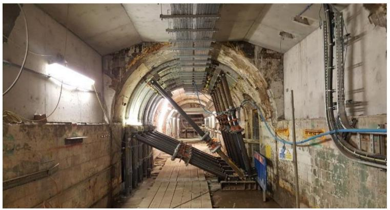
Innovative temporary & permanent masonry tunnel support shown in temporary support condition prior to formation of new opening
