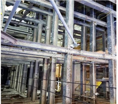
Temporary works were detailed for flexibility, simplicity, speed & safety Holistic approach allowed recovery of temporary works members for re-use
