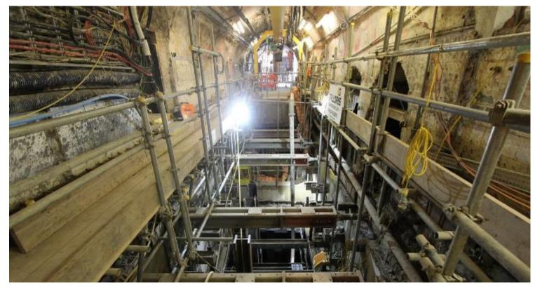
Underpinning of distressed dis-used passageway between the two Underground Platform tunnels to allow new opening and undermining to form a new access to new lift shaft
