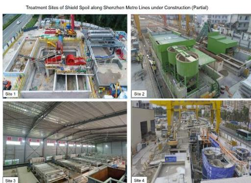
Shenzhen Metro Line 14 features an overall distance of 50.34 km, connecting Futian District with Pingshan District. A group of 49 TBMs have been employed for the tunneling work, adopting earth pressure balance shield method. The process of shield tunneling produces massive shield spoil containing sand, stone, gravel, clay, water, shield additives, etc. Due to its high moisture and weak mechanical properties, shield spoil has commonly been regarded as waste. Traditionally, shield spoil is shipped
