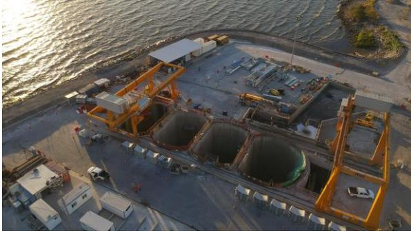
The “Desarrollo Sustentable de la Cuenca Matanza-Riachuelo - Lot 3” project includes a gravity outfall system to discharge treated wastewater into the River Plate, in Buenos Aires (Argentina). It consists of: 50 m deep upstream shafts; 10.5 km long sub-fluvial outfall tunnel; 1.5 km long diffuser tapered tunnel; 34 risers to discharge the effluent from the diffuser tunnel up to the river bed
