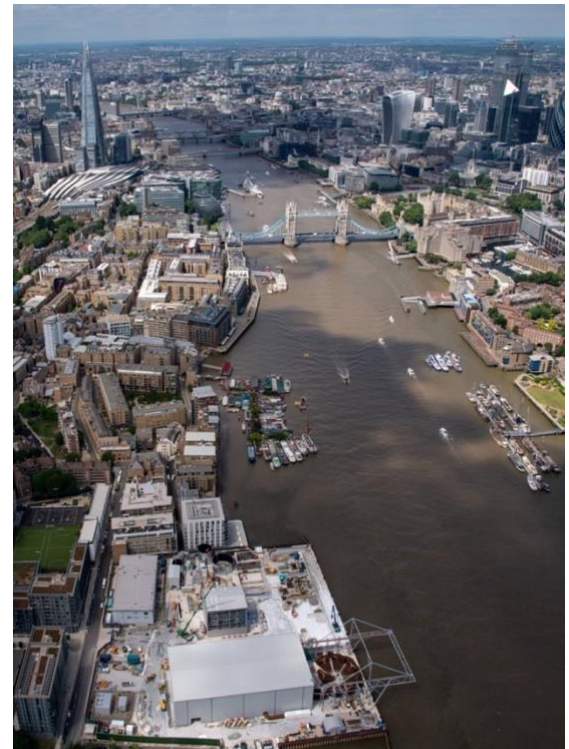
Riverside construction site of Major Project Award Winner, Thames Tideway in London, UK
